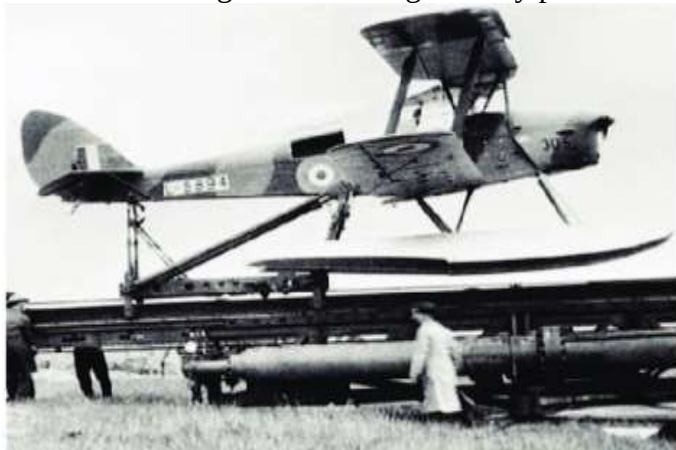
Figure 1. The first multi-role flying target, the de Havilland DH.82B Queen Bee
