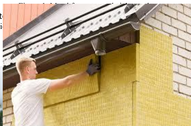
Figure 4. Basalt-wool insulation combined with a ventilated façade
